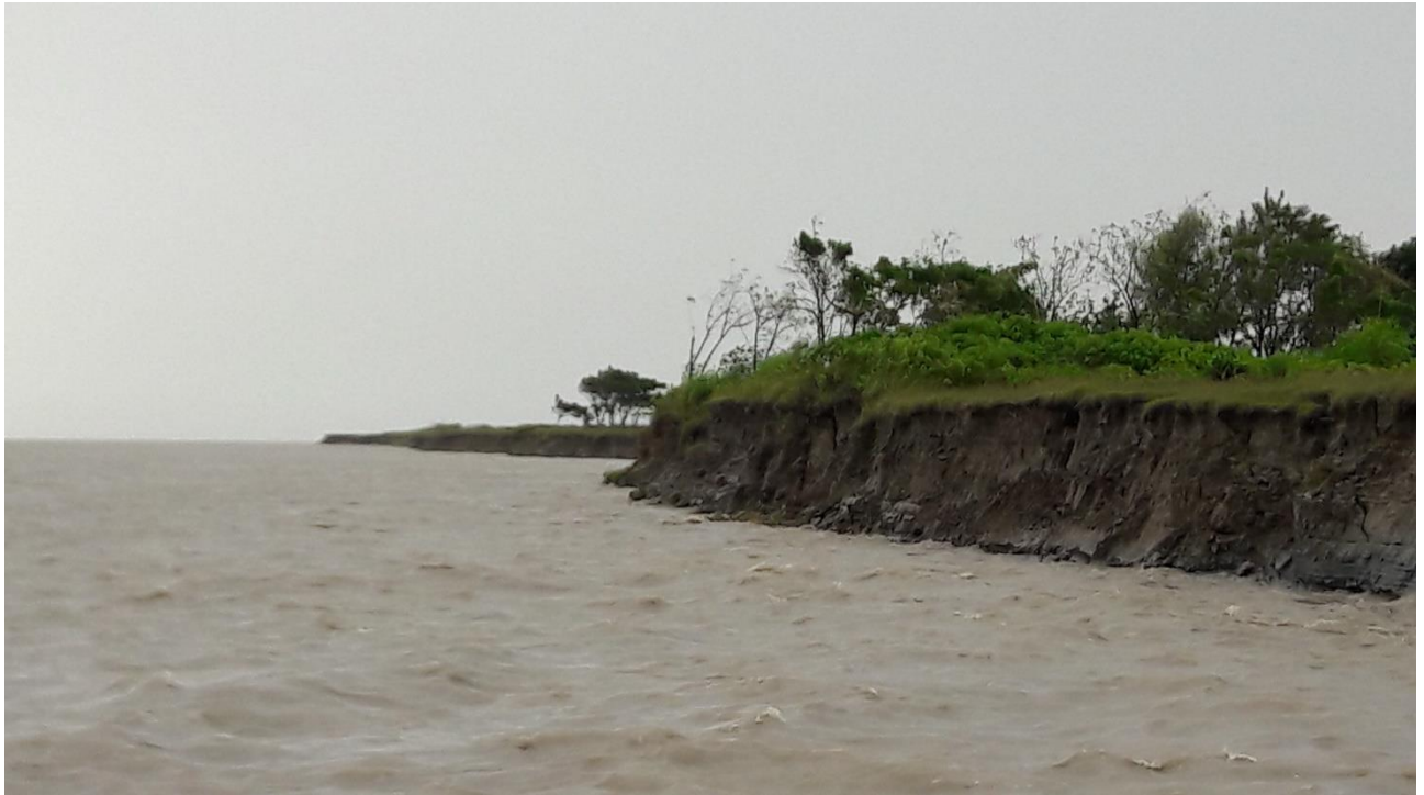
Figure 1.4 View of the western shoreline of the Gulf of Mottama (29 September 2018; near An Lan Pya). The steep, nearly vertical bank and the slumped blocks are evidence of the main erosional mechanism of the bank (slope collapse) that results from the ongoing landward migration of the tidal channel.
