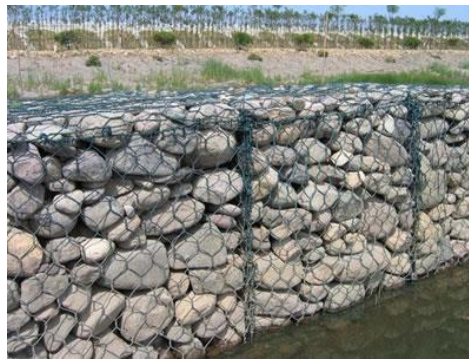
Gabion Mesh Boxes
